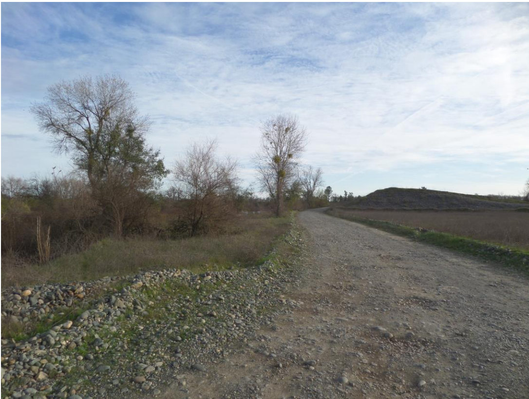
Photo 18: View of existing inflow weir, looking south.
