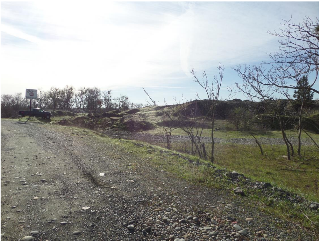
Photo 2: View of southern parking lot regrade area, looking southwest.
