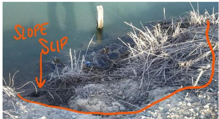
LS view: section of levee has slipped at pipe crossing.
