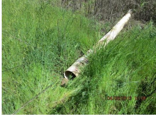
WS-a disconnected pvc pipe on levee slope
