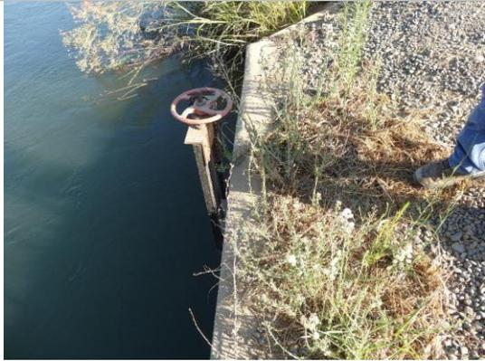
LS view: screw gate and concrete headwall visible on LS.
