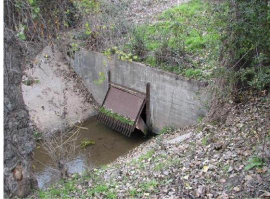
Concrete headwall and flap gate on WS toe.
