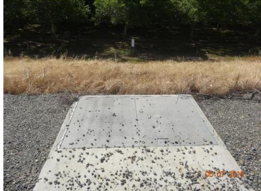
WS view: concrete vault with cover and paddle marker visible on WS pipe alignment.
