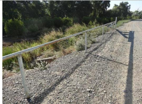
WS view: guardrail along the WS slope and concrete headwall visible on WS.
