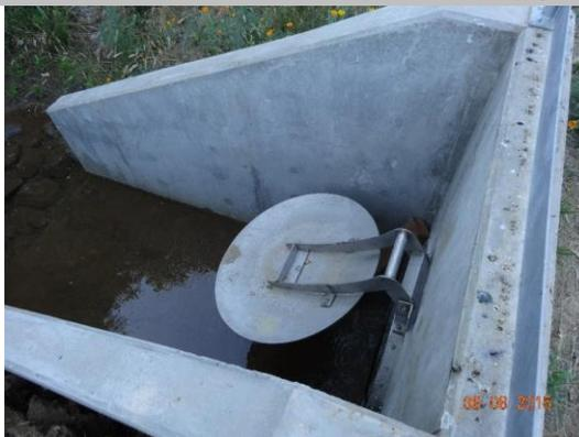
WS concrete headwall and flap gate.
