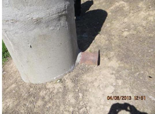
LS- concrete standpipe with disconnected steel pipe
