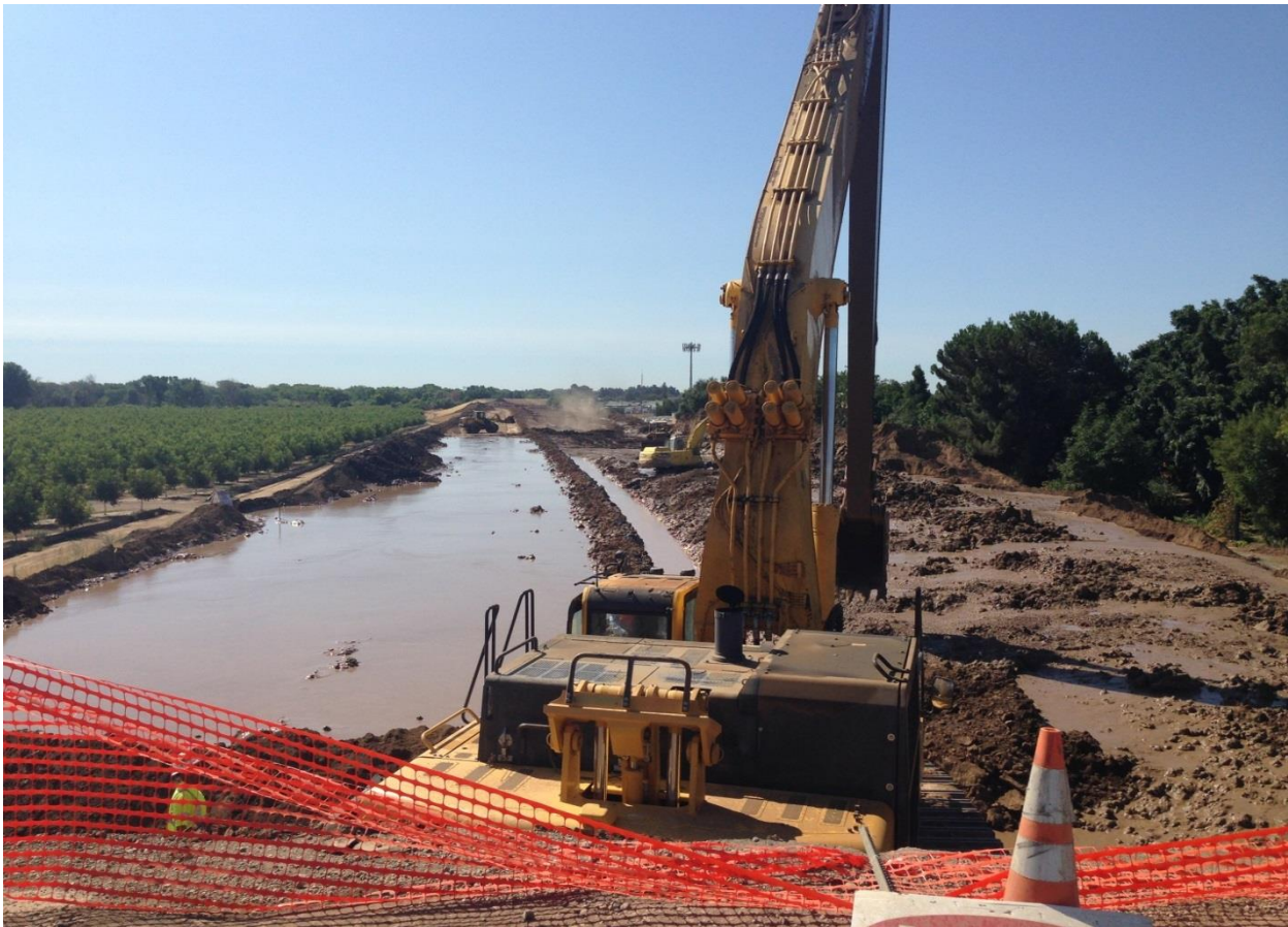
Feather River West Levee Project Source: Sutter Butte Flood Control Agency
