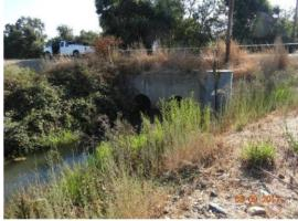
LS view: concrete headwall with dual 60-inch crossings visible from LS.
