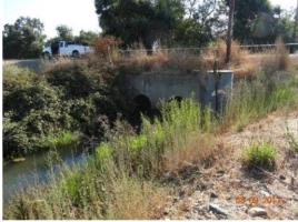
LS view: concrete headwall with dual 60-inch crossings.
