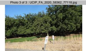
Overview of LS at crossing. Markers along pipe alignment indicating pipe depth of 4-feet (near levee shoulder) and 3-feet near toe.
