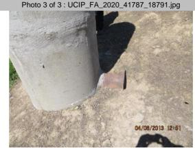
LS- concrete standpipe with disconnected steel pipe
