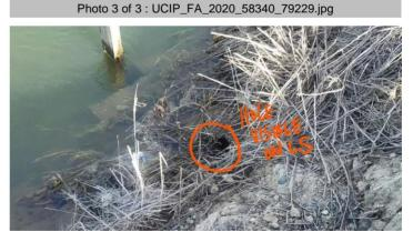
LS view: hole visible on LS, appears to be linked to burrow hole that is allowing flow to go into pipe.
