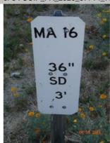
WS marker indicating location and depth of pipe through slope.
