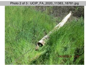
WS-a disconnected pvc pipe on levee slope
