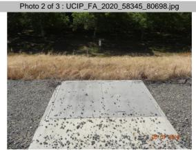
WS view: concrete vault with cover and paddle marker visible on WS pipe alignment.
