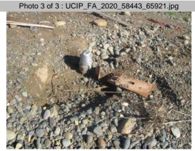
Photo 1 of 2. View of localized erosion at air vent located on WS shoulder.
